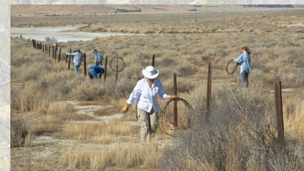
These volunteers braved the heat to remove relic fencing from the Carrizo! Photo by Bryant Baker
