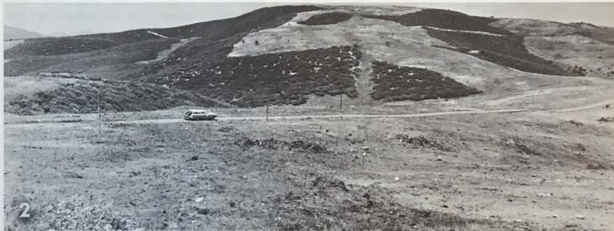
NO. 2.--Same area one year after removal of heavy brush from selected areas suited to type conversion. Fire hazard is greatly reduced and control of wildfire facilitated.
