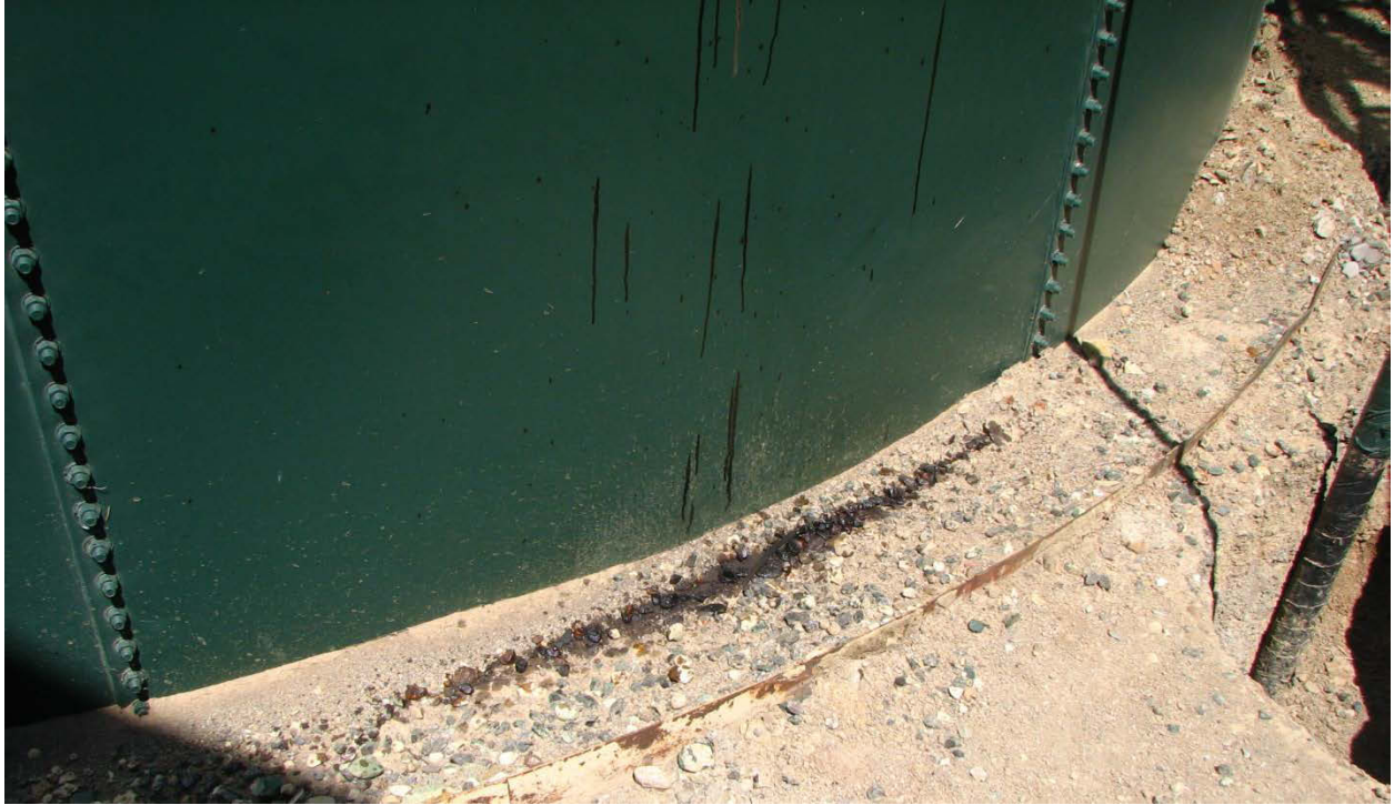
Crude Oil Tank 8 has a small oil leak, with oil accumulating at its base that could present a hazard to condors and other wildlife.
